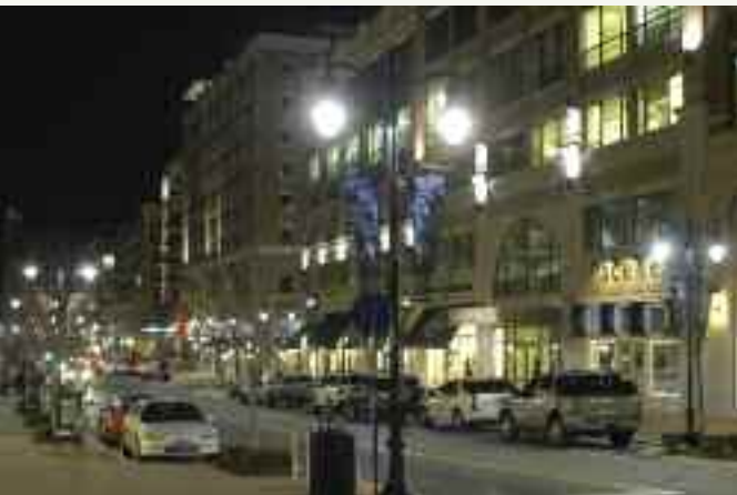
PHI's Pilot LED Streetlight Project is testing customer response to the newly developed fixtures, as well as their reliability, energy efficiency and light quality. In addition to their energy savings, the LED lights are directional, so they don't cause "light pollution" in our night skies. The first of PHI's test LED streetlights were installed at National Harbor in Prince George's Co., Md.
